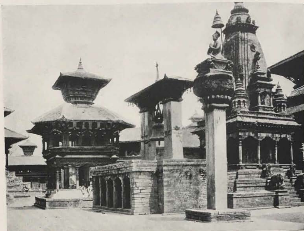
TEMPLE IN BHATGAON SHOWING SEATED FIGURE OF BHUPATINDRA MALL, IN BRONZE ON CARVED PILLAR AND FINE BRONZE BELL
